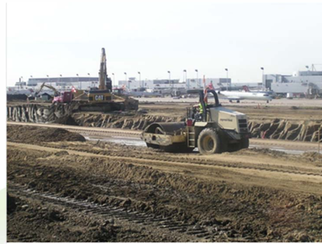
Construction at MSP MPR Photo/Dan Olson
