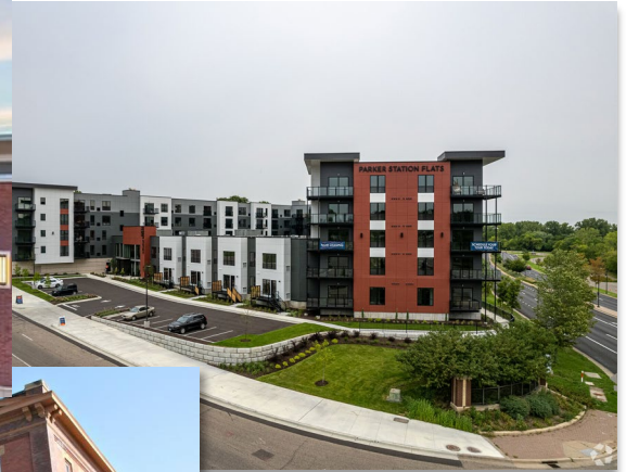
Parker Station Flats Robbinsdale, MN
