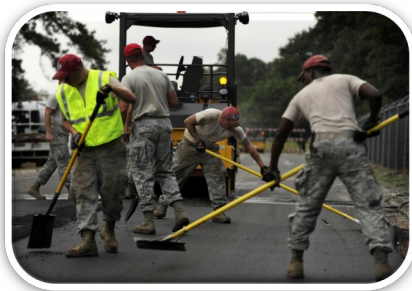
Road Reconstruction Projects
